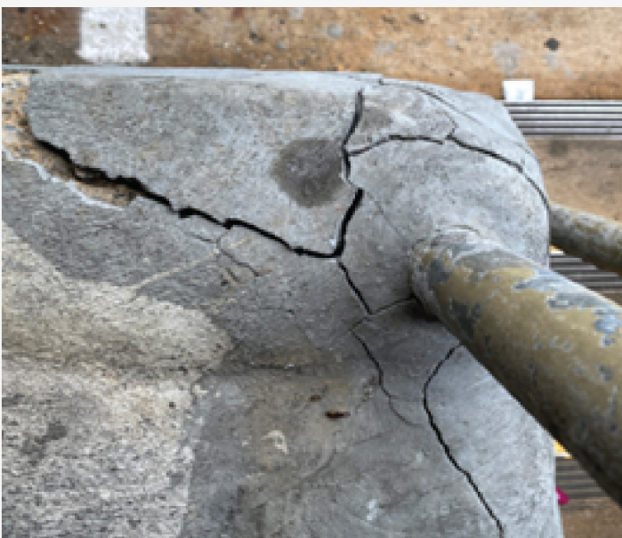
Figure 11. Cracked Concrete
